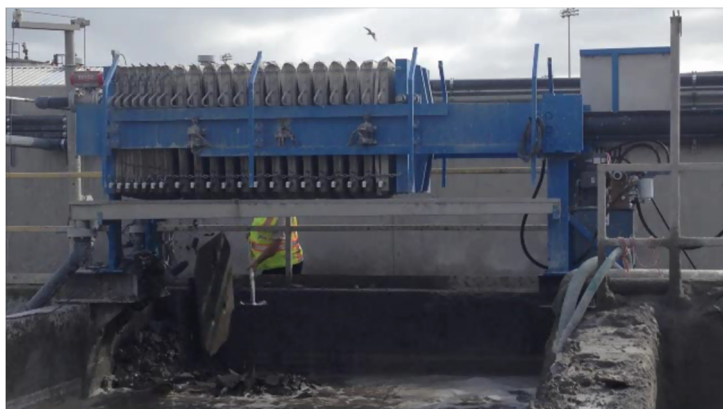
Below: Temporary installation I-beam frame over pit
