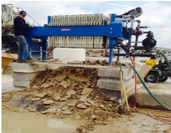
Above: Temporary installation on blocks
